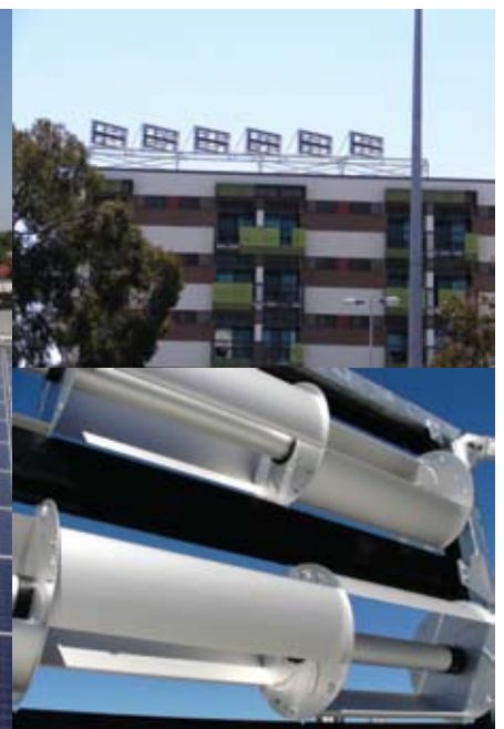
St. Bartholomews, Perth, Western Australia. 6kW roof top installation on a residential and office building. Turbines have been oriented to face the prevailing wind to ensure the highest return. Windpods and solar PV can work hand in hand, as the sun and wind resource are not cross-effected in any way. In northern hemisphere regions with low sun-hours, Windpods can be particularly effective.
