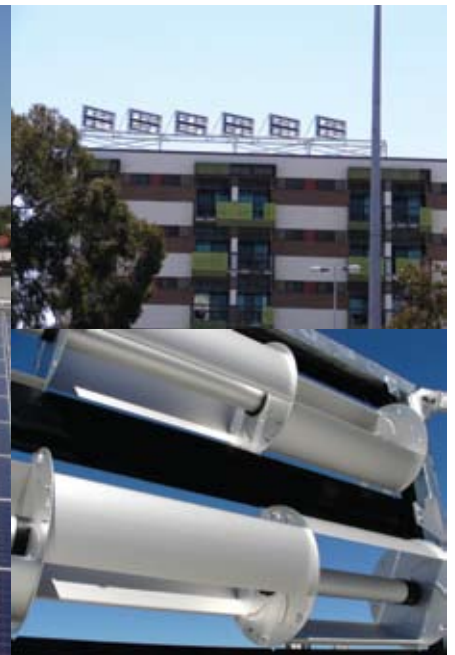
St. Bartholomews, Perth, Western Australia. 6kW roof top installation on a residential and office building. Turbines have been oriented to face the prevailing wind to ensure the highest return. Windpods and solar PV can work hand in hand, as the sun and wind resource are not cross-affected in any way. In northern hemisphere regions with low sun-hours, Windpods can be particularly effective.
