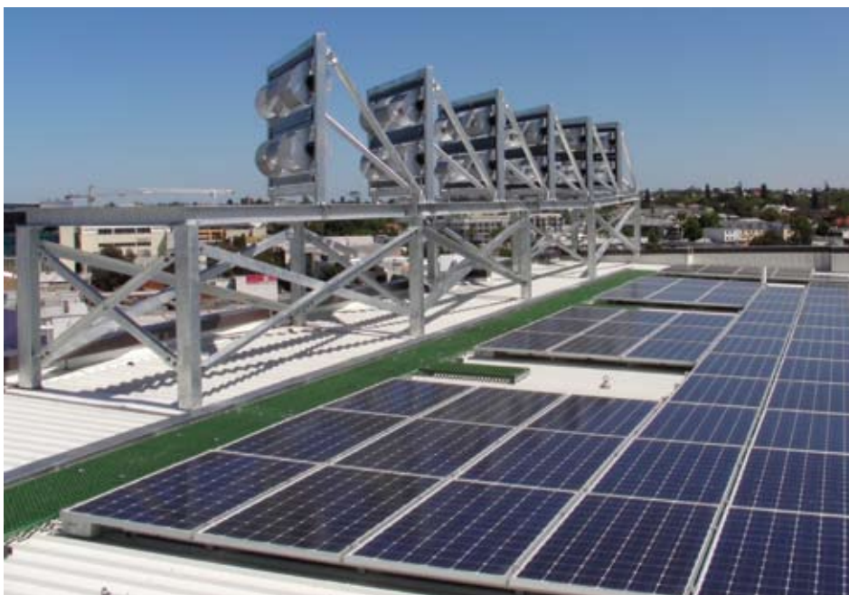
St. Bartholomews, Perth, Western Australia. 6kW roof top installation on a residential and office building. Turbines have been oriented to face the prevailing wind to ensure the highest return. Windpods and solar PV can work hand in hand, as the sun and wind resource are not cross-effected in any way. In northern hemisphere regions with low sun-hours, Windpods can be particularly effective.
