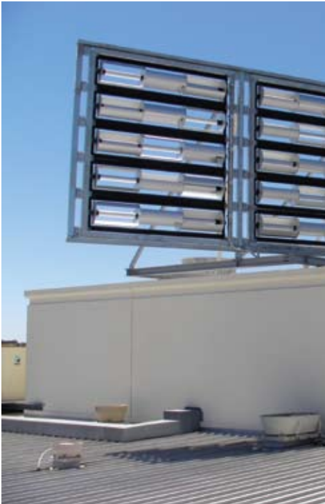
City of Cockburn, Perth, Western Australia. 10kW installation of Windpods, mounted on top of a services room on the rooftop. The footprint of this 10kW Windpods is similar to 2.5kW of solar PV. Also see the inverter bank, switchboard and brake system (to the right of the switchboard), all located undercover in the services room. The switchboard has a manual over-ride for the brake system for high wind alerts or maintenance and servicing.
