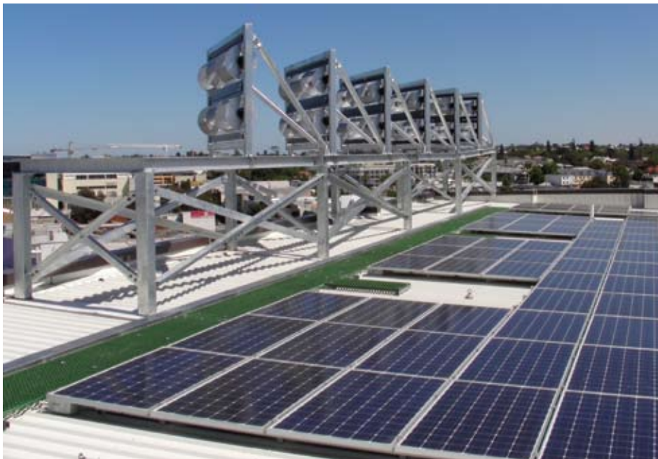
St. Bartholomews, Perth, Western Australia. 6kW roof top installation on a residential and office building. Turbines have been oriented to face the prevailing wind to ensure the highest return. Windpods and solar PV can work hand in hand, as the sun and wind resource are not cross-affected in any way. In northern hemisphere regions with low sun-hours, Windpods can be particularly effective.
